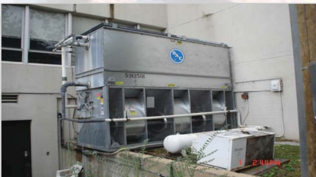
Cooling Tower Condition
