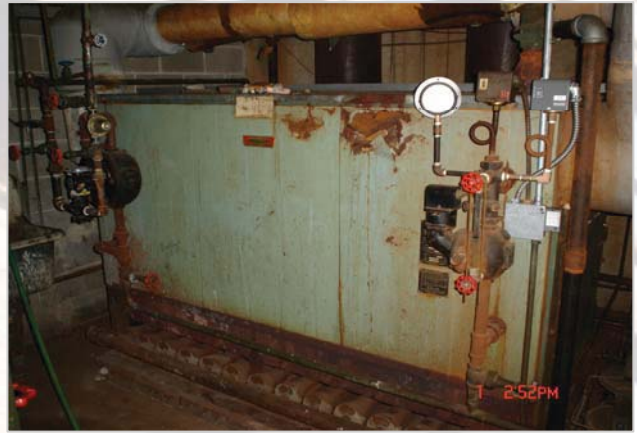
Assessment of Expected Useful Life (EUL), deteriorated condition that may require replacement
