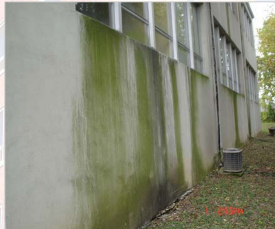
Condition of exterior finishes
