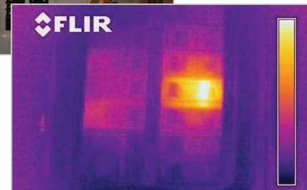
**Electrical and Fire Hazard Problems:** It was noticed during a commercial inspection of an office/warehouse that lights were flickering when other lights were turned on. *By looking at the electrical distribution panel we were able to easily spot the problem circuit.* Further investigation revealed that the circuit breaker was undersized for the intended application and was double tapped. This presented a fire hazard and shock hazard.
